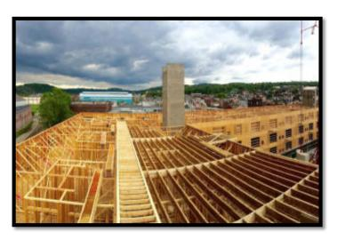
The second through the sixth floors were analyzed during this technical report. The first floor is concrete for the parking garage and was omitted from this analysis. As seen above in the wall section the building has wooden framing this is typical for the second through eighth floors. It was natural to explore metal framing as a structural system to replace the wooden framing. The relative quickness and cost of the wooden frame is the reason why this structural system was chosen.
